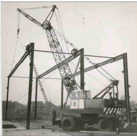
1972: Rope-driven SK 15 with plastic operator cab
